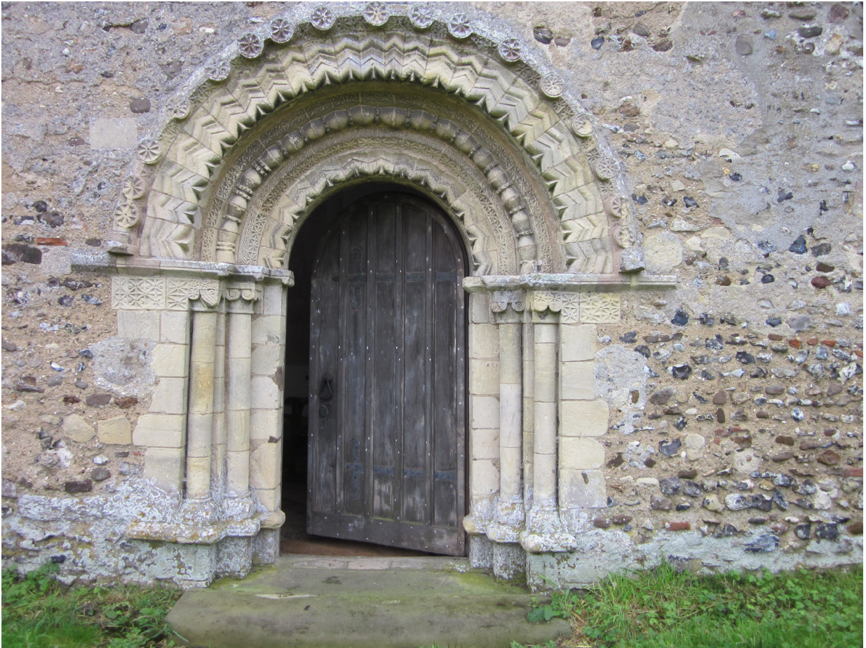
Figure 1.12. The Norman north nave door at Hales Church, Norfolk (TM 383 960). Note all stone carving occurs on the relatively smooth bedding plane surfaces of stones which face to the north (or BVEIA).
