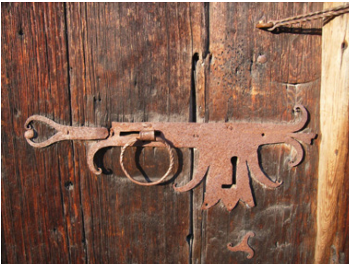
Figure 1.6. A pull-ring lock Swedish key (dated to 1312-1313) photographed by Dr R. Borg. The mechanism requires two hands operate - one to draw the bolt, the other to turn the key.
