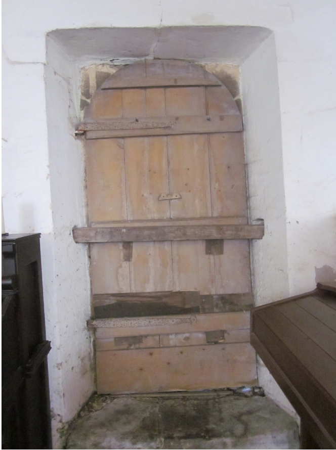
Figure 1.7. The north aisle door at Stragglethorpe, Lincolnshire (SK 913 524) which is retained in position by a bar lock.
