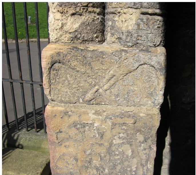
Figure 1.13. At Monkwearmouth, Durham (NZ 402 577) the Anglo-Saxon sea-bird carvings related to the west doorway can be seen on the relatively smooth bedding plane surfaces in the north jamb, and therefore on stones orientated BVFIA.
