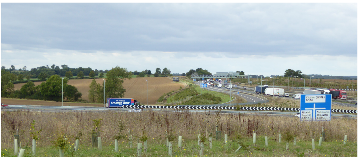
Fig 1.13 View looking north-west from Harlington Road, Toddington, after completion
