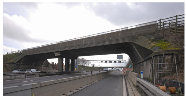
Fig 1.17 The Chalton overbridge before demolition, Site R, looking south-east
