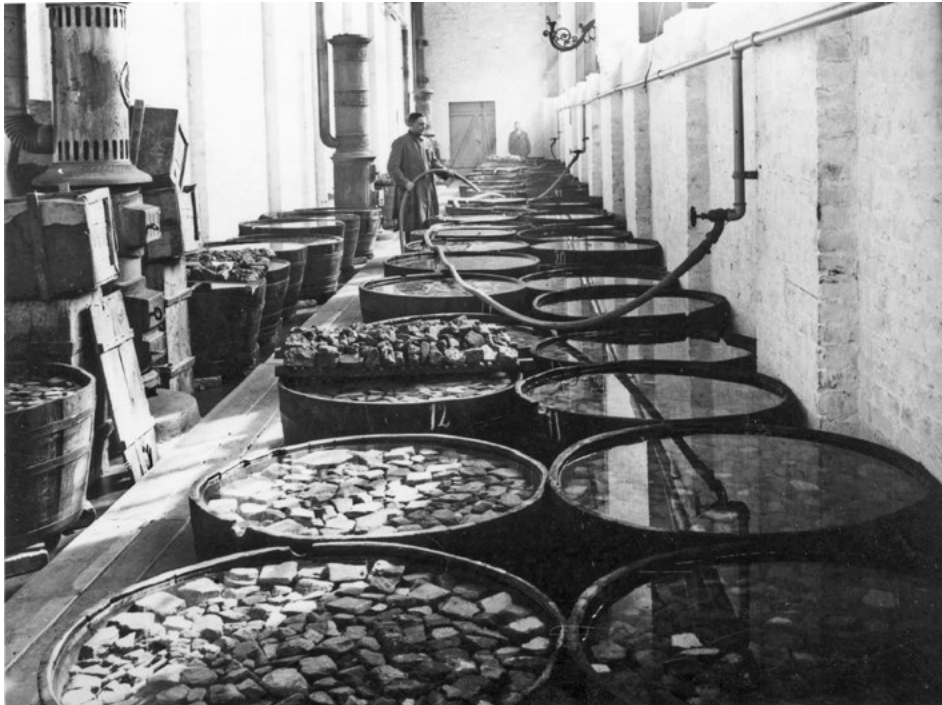
Figure 1. Ishtar Gate fragments in the 1920s, VA. Cleaning glazed bricks fragments from salts. PhBab 3701 (© Vorderasiatisches Museum, SMB).
