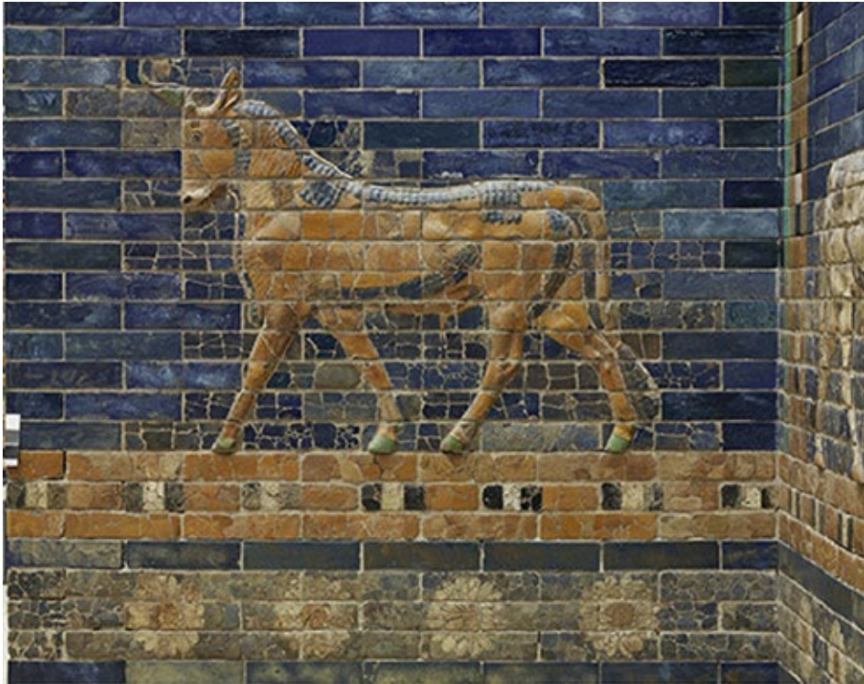
Figure 12. Ishtar Gate, glazed bull relief. VAM reconstruction. The bull and the decorative band below were assembled with ancient brick fragments, whereas the complete bricks in the background are modern. 45 relief bricks were required for each bull. The bull is 1.1 m high (© Vorderasiatisches Museum, SMB, photo: Olaf M. Teßmer).
