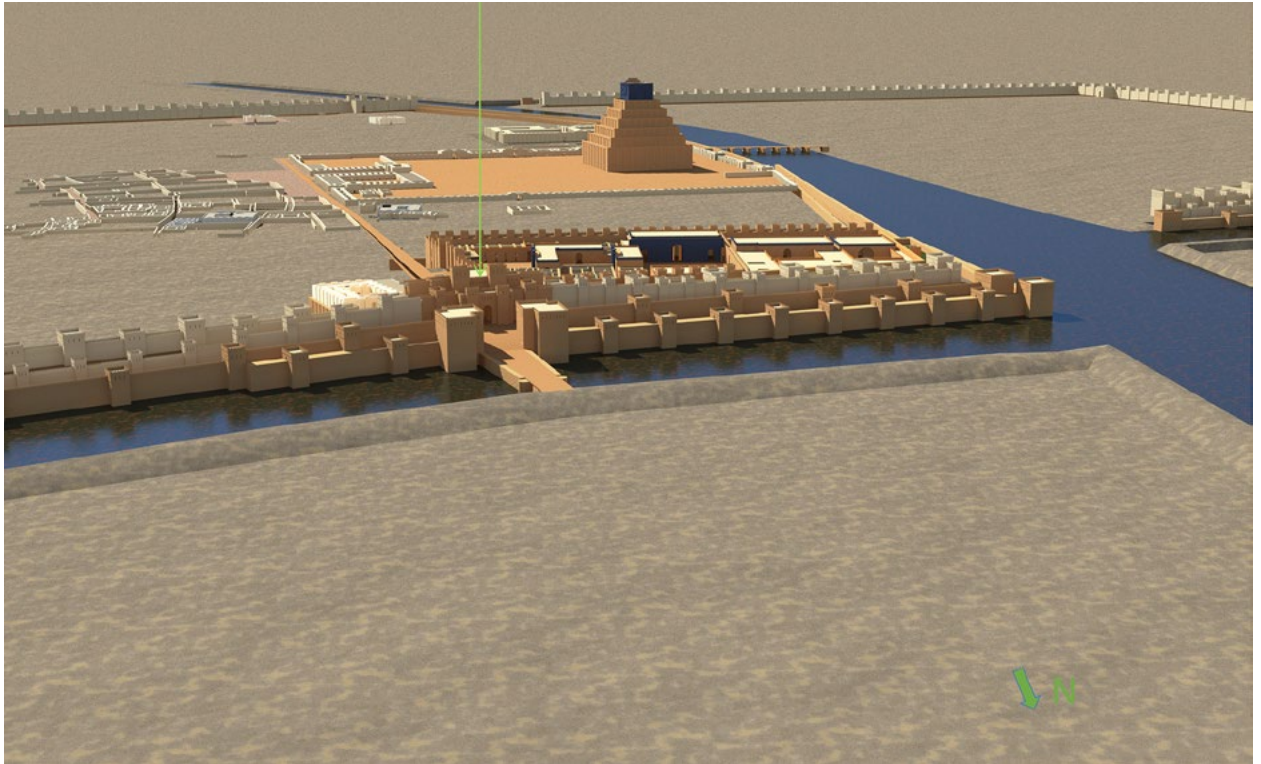
Figure 22. Babylon digital model looking south. Ishtar Gate during early reign of Nebuchadnezzar II (604–562 BC). Reliefs of unglazed bulls ( rīmu ) and dragons ( mušḫuššu ) on the gate walls. Reddish-brown walls are baked brick and whitish-grey walls are unbaked mudbrick in all model pictures.
