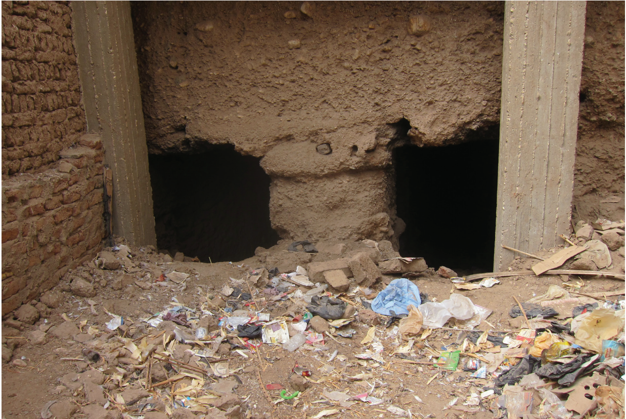
Figure 6. Concrete pillars erected outside the façade of Saff el-Kissasiya royal tomb (photo R. Soliman, January 2017).
