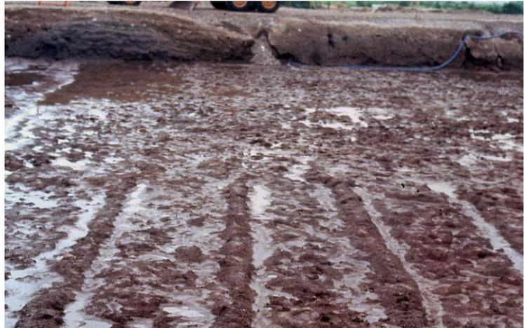
FIGURE 10 VERTICAL BUNDS UNDER CONSTRUCTION AT ARIMA-JŌRI
