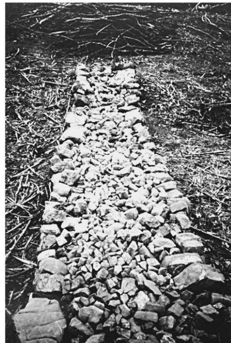
Newly-constructed silt-trap terrace on a Copan hillside. Fig. 19
