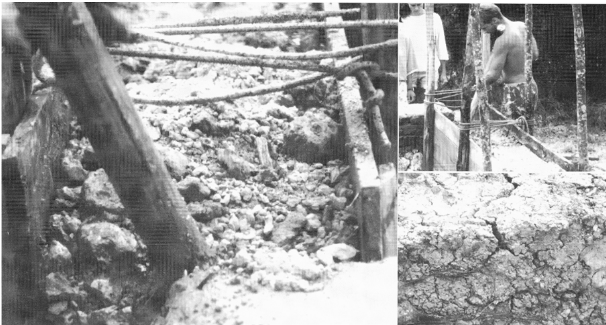
FIGURE 5.8. THE CONSTRUCTION OF PISE WALLS AT ALLUMIERE USING TRADITIONAL TECHNIQUES (GENOVESI 2001: FIG. 2, P. 314), COURTESY OF THE EDITORIAL COMMITTEE OF THE SWEDISH INSTITUTES AT ATHENS AND ROME.
