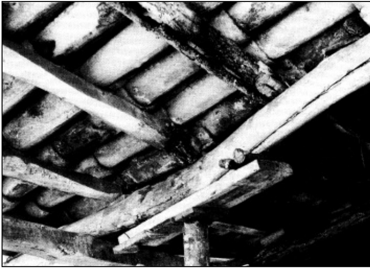
FIGURE 5.21. PHOTO (TAKEN 1991) OF A MODERN TILED ROOF WITH TILES RESTING DIRECTLY ON THE RAFTERS (WIKANDER 1993: FIG. 50, P. 123), COURTESY OF THE EDITORIAL COMMITTEE OF THE SWEDISH INSTITUTES AT ATHENS AND ROME.
