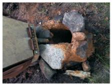
5 - Constructing of the furnace. Granite blocks are put with the use of clay mortar.
