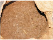
Heaving of the clay lining on the bottom in the process of drying. Therefore in the process of drying it was necessary to seal the surface.
